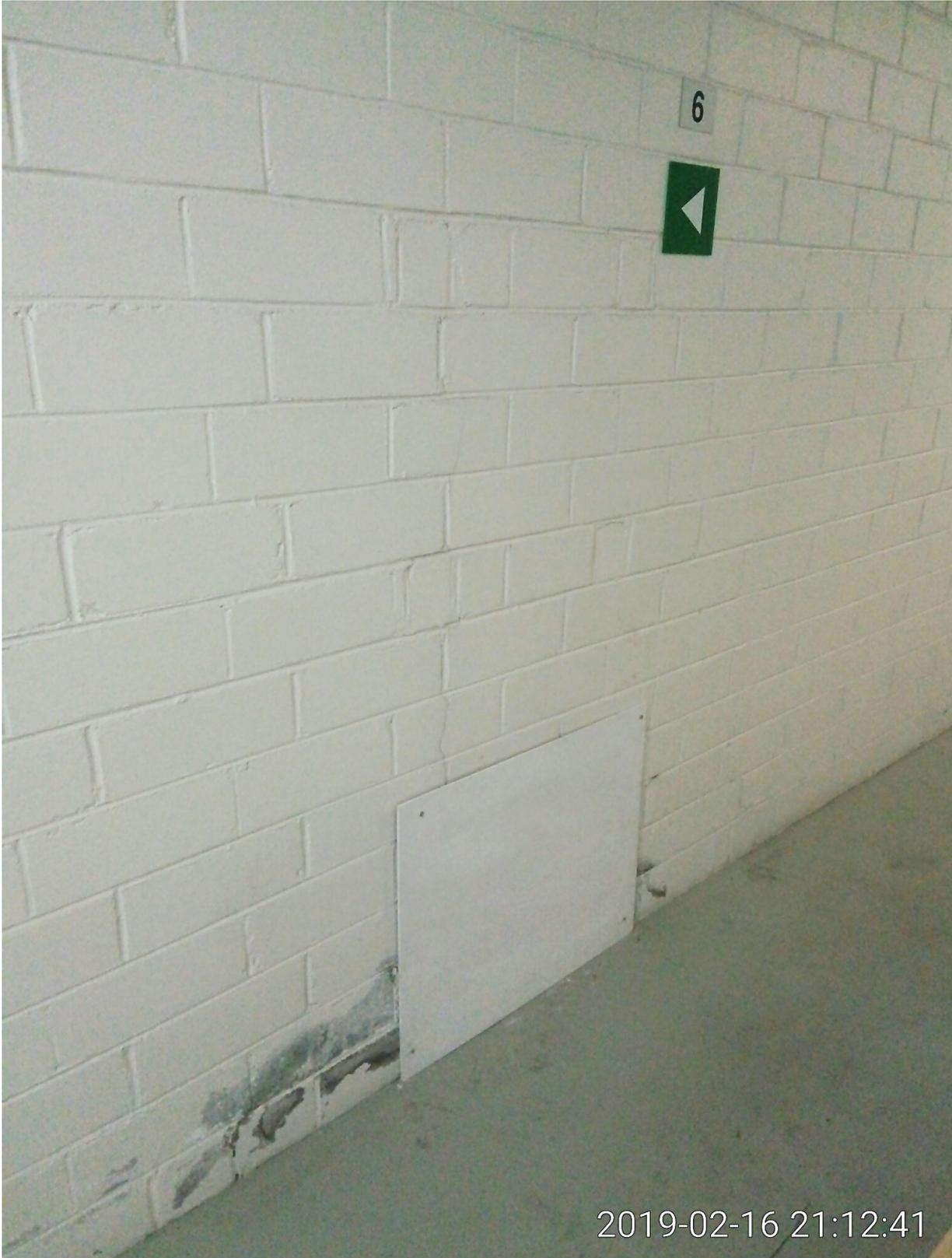
SP52948 Block C Level 6 large hole in wall simply riveted by large panel and no further repairs occurred on 1<sup>st</sup> of March 2019
