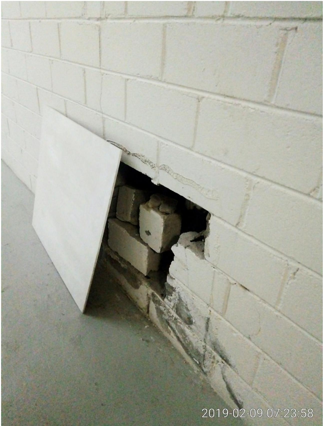
SP52948 Block C Level 6 large hole in wall simply riveted by large panel and no further repairs occurred on 16<sup>th</sup> of February 2019
