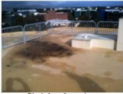
Block A roof coverings
