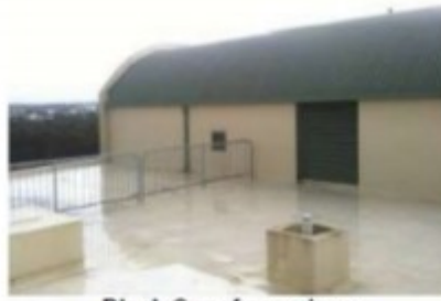
Block C roof coverings
