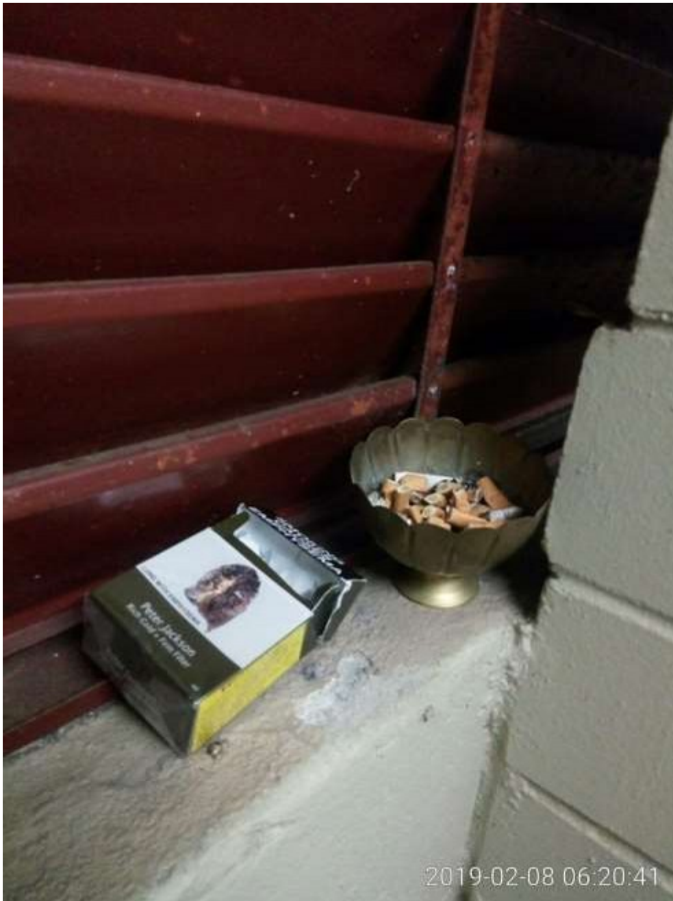
Example of hiding cigarette butts near louvres behind fire door 2 below Block A in February 2019:
