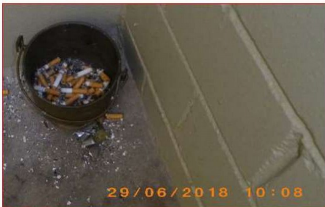
Examples of smoking near fire door 2 below Block A in June and July 2018:
