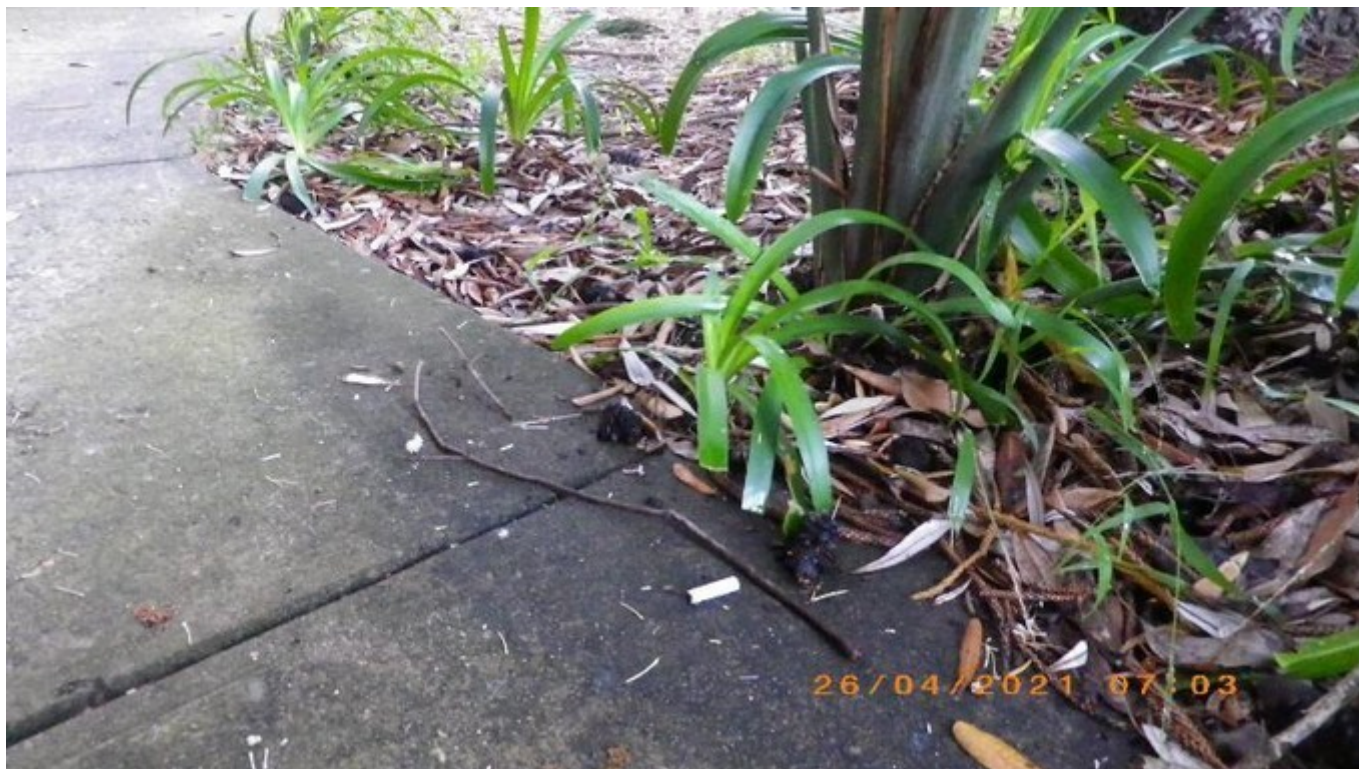
17 Smoking in the complex continue to be a serious fire safety risk – Block D garden pathway where lot of dry barks and leaves cover the grounds
