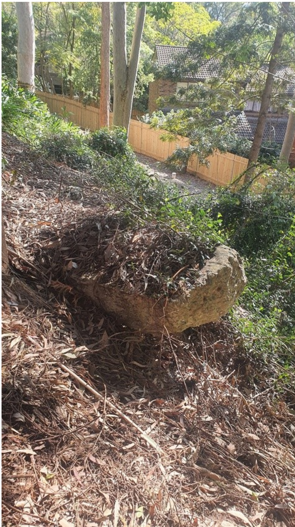
54 Large piece of concrete slab at risk of rolling down eroded soil behind townhouses – unattended for more than seven years as of 1 st of October 2021
