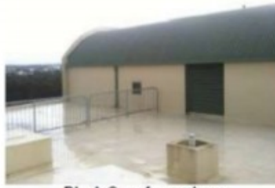
Block C roof coverings
