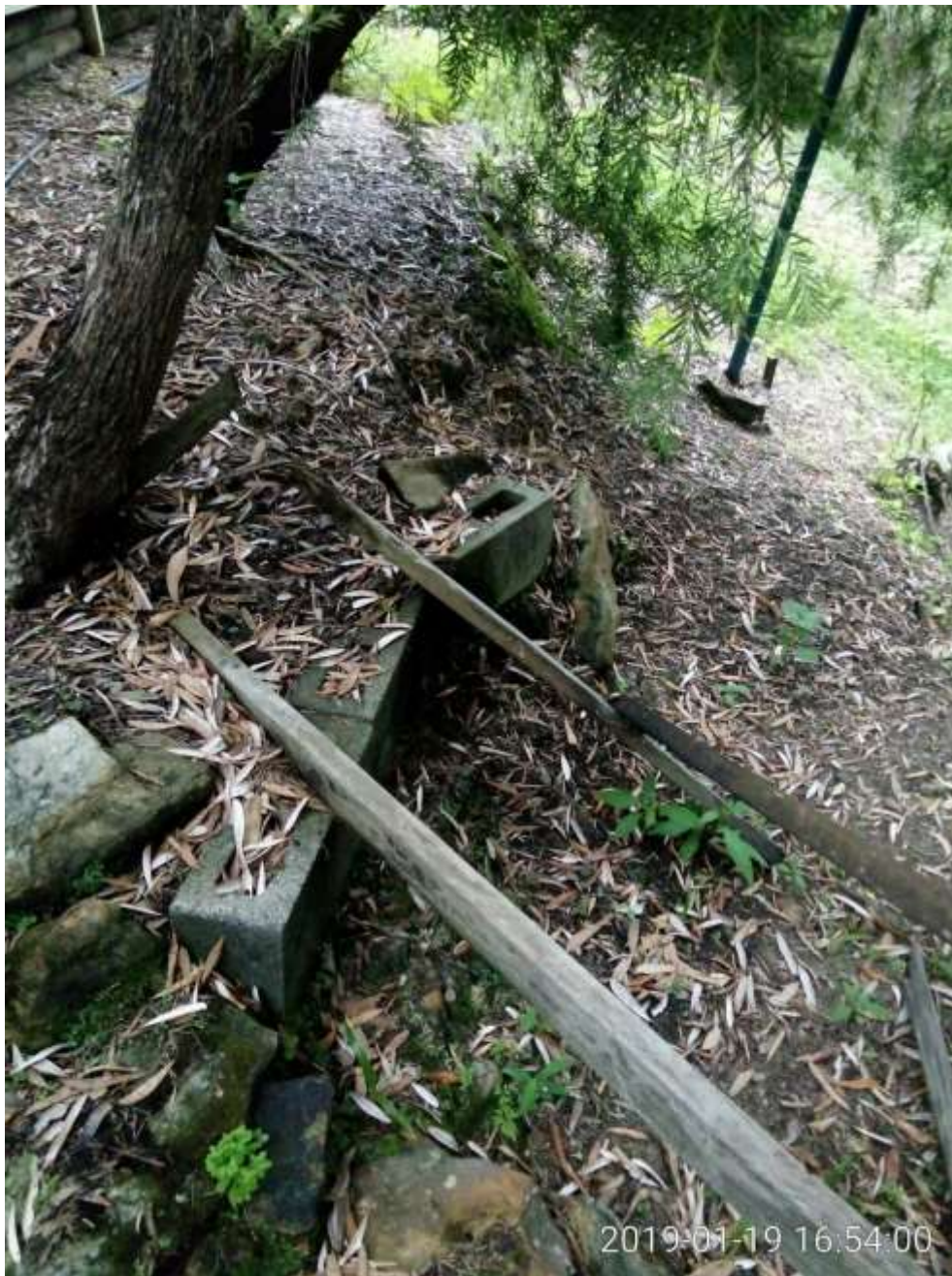
SP52948 – Collapsed wooden railings behind townhouses on 19 th of January 2019
