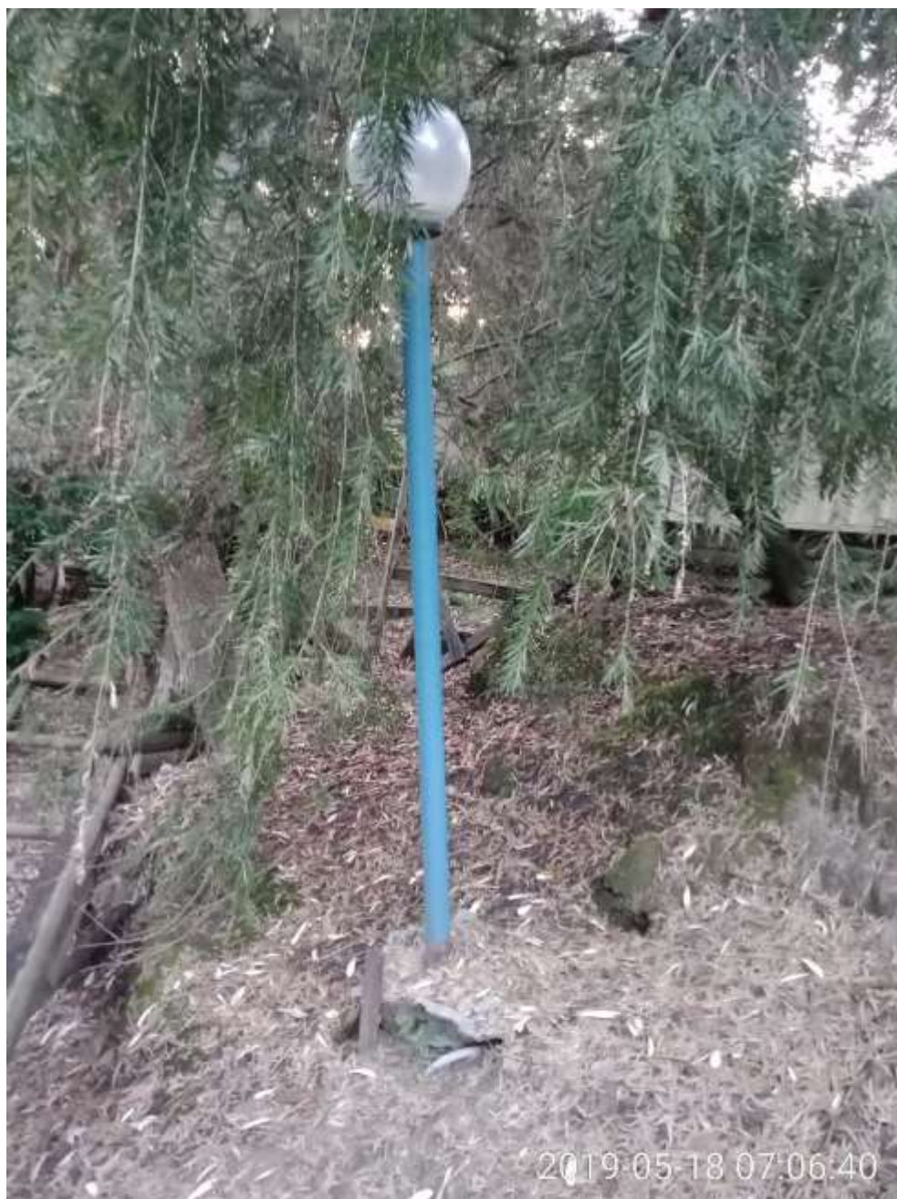
SP52948 Light pole behind townhouses on unsafe grounds due to eroding soil
