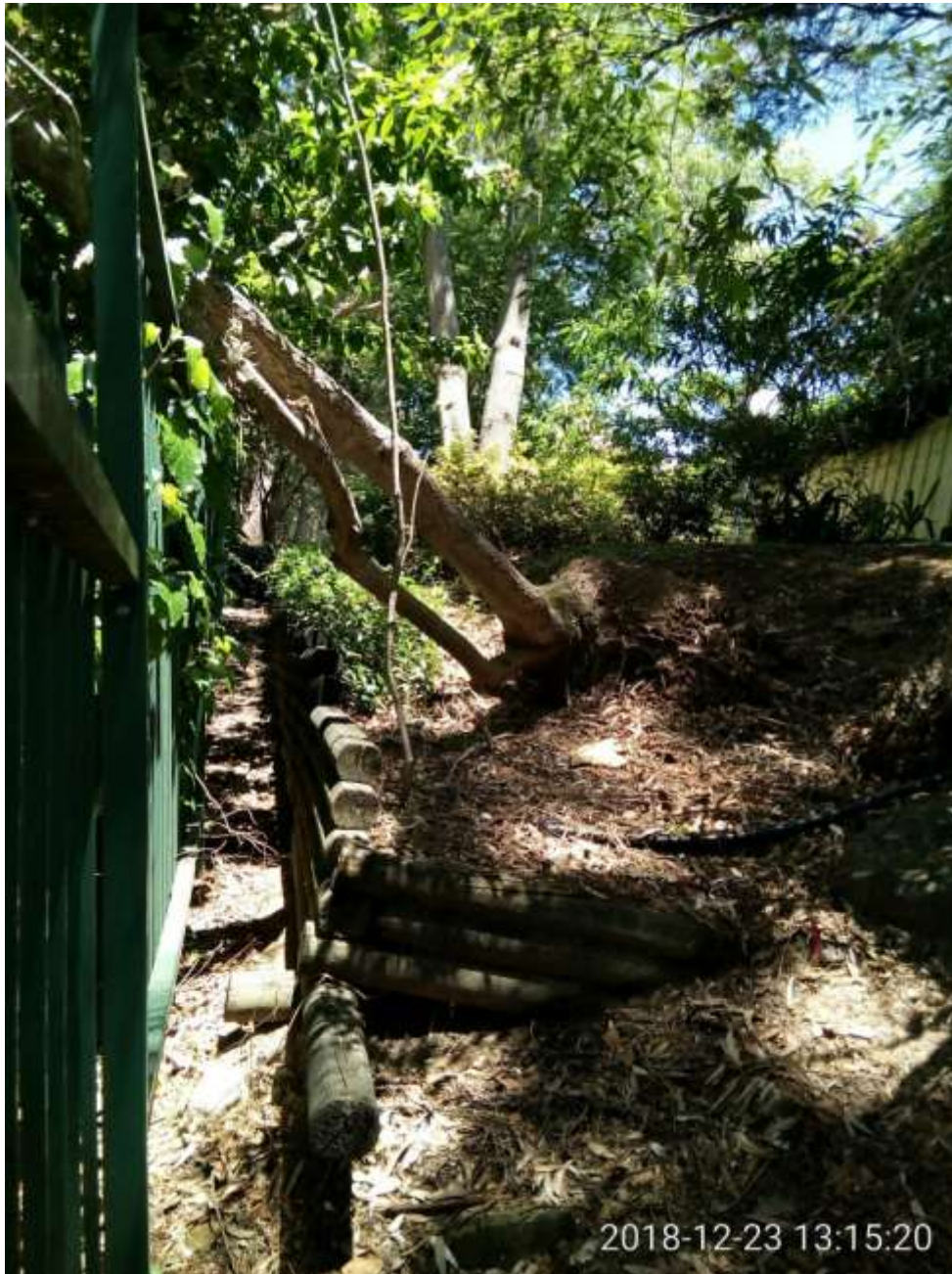
SP52948 Unsafe slope due to eroding soil and unrooted tree behind townhouses towards Fontenoy Road – photos taken in period 23 rd of December 2018 to 18 th of May 2019
