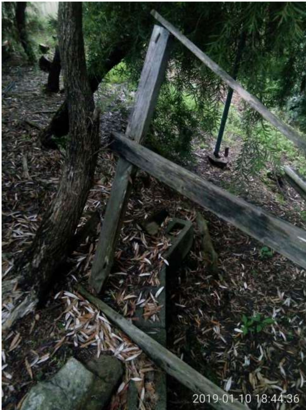
SP52948 – Unsafe rotten wooden railings behind townhouses on 10 th of January 2019
