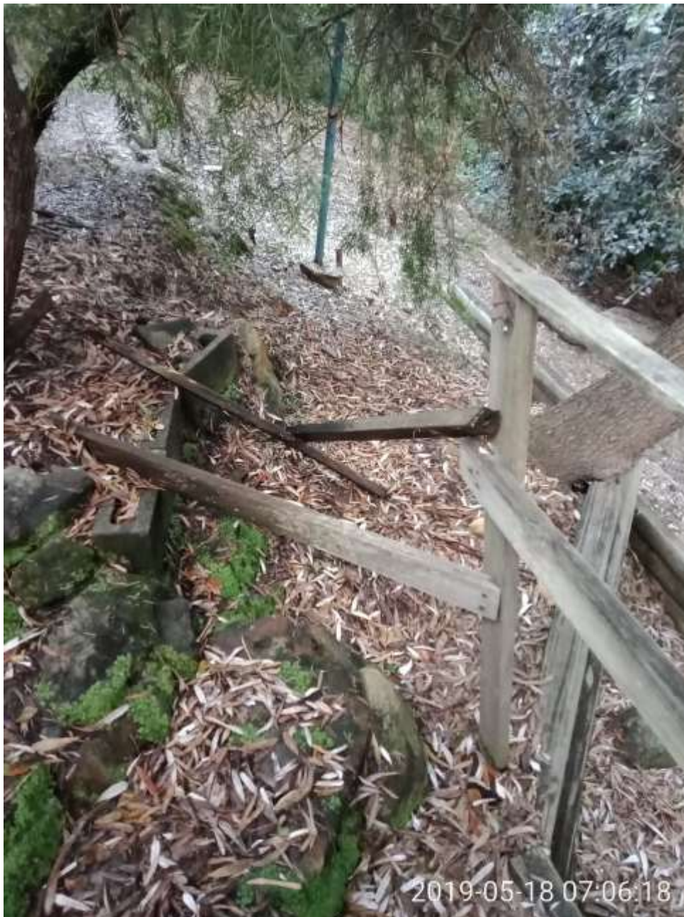
SP52948 – Collapsed wooden railings behind townhouses on 19 th of May 2019
