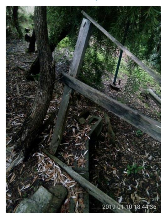
SP52948 – Collapsed wooden railings behind townhouses on  $19^{\text{th}}$  of January 2019
