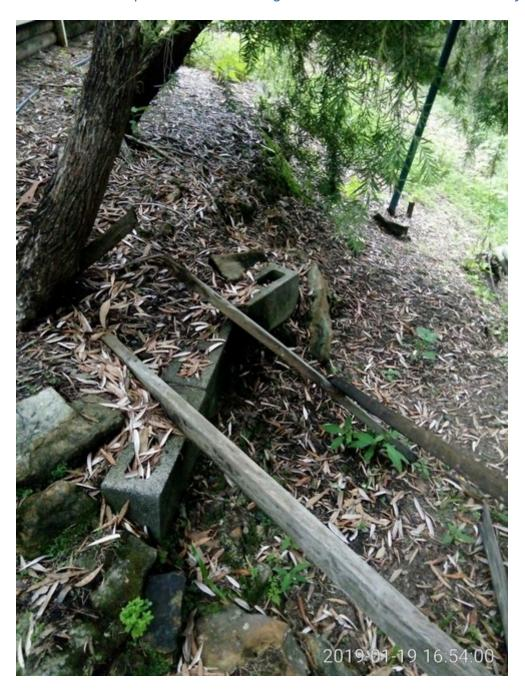
SP52948 – Collapsed wooden railings behind townhouses on 30<sup>th</sup> of January 2019
