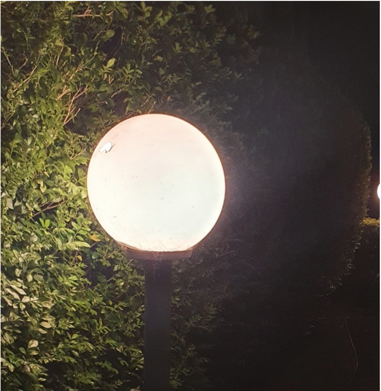
SP52948 – damaged light post globe in garden near Block D on 19 th of October 2021
