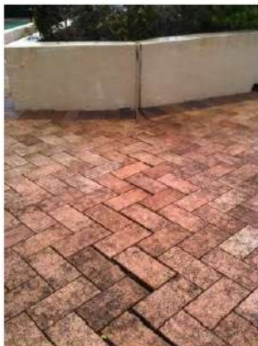
Isolated raised paving
