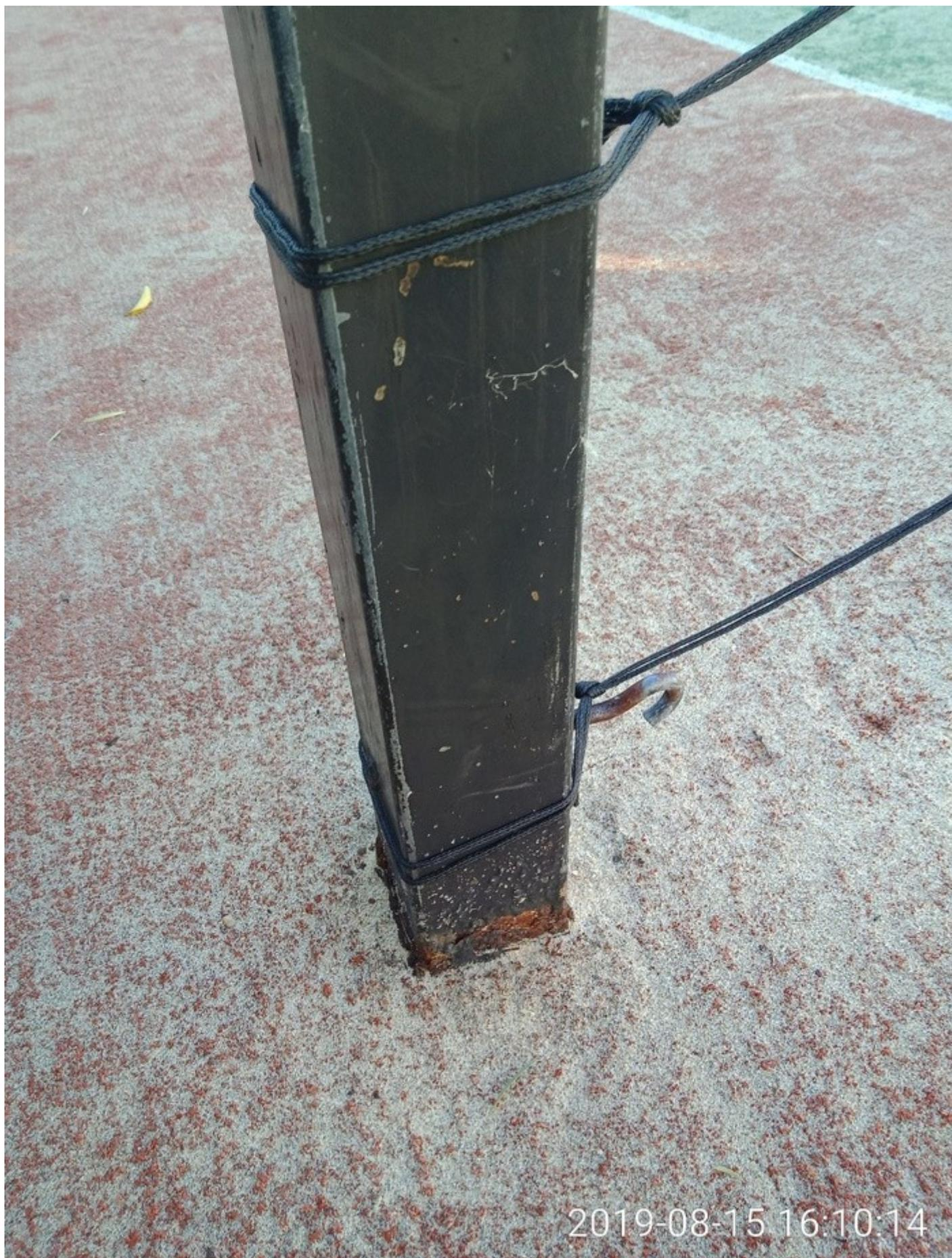
SP52948- Examples of tennis court fence damages and sharp wires protruding that caused scratch injuries to female owner on 15<sup>th</sup> of September 2019
