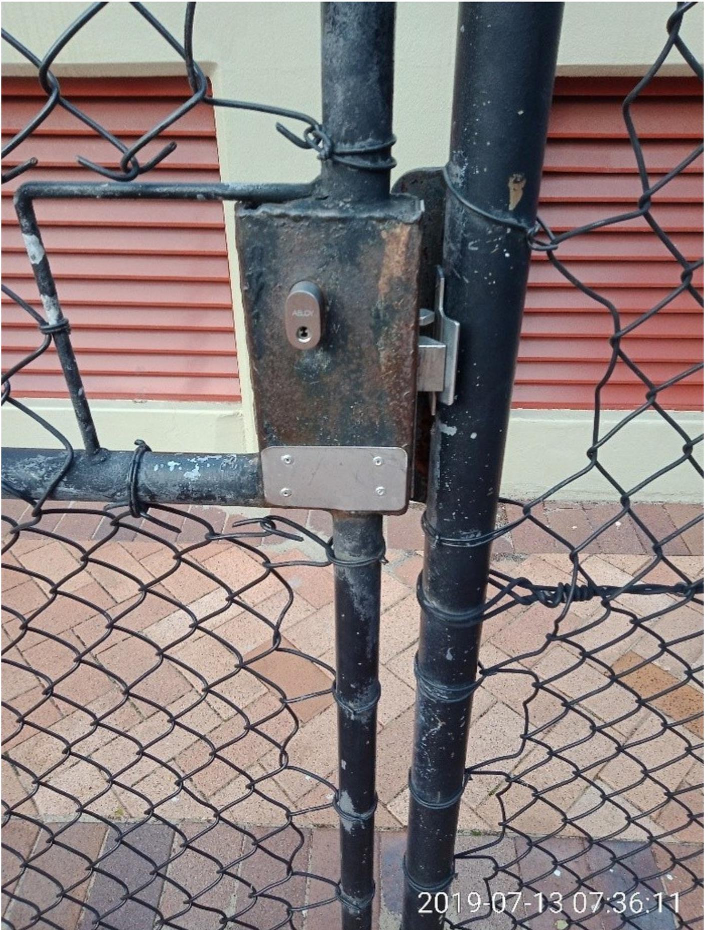
SP52948- Rusted lock on tennis court - paint after second owner's complaint about incomplete repair - 11<sup>th</sup> of August 2019
