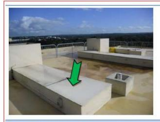
Photo 1. Block A, roof, box covers – non-asbestos containing compressed fibre cement panels
