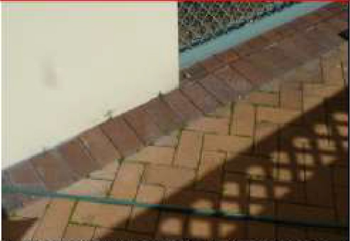
Note height of pavers in relation to weep holes for unit 151
