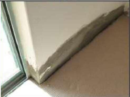
Poorly carried out and unfinished internal render repairs within unit 150
