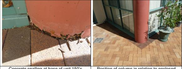
Concrete spalling at base of unit 150's enclosed patio area column
