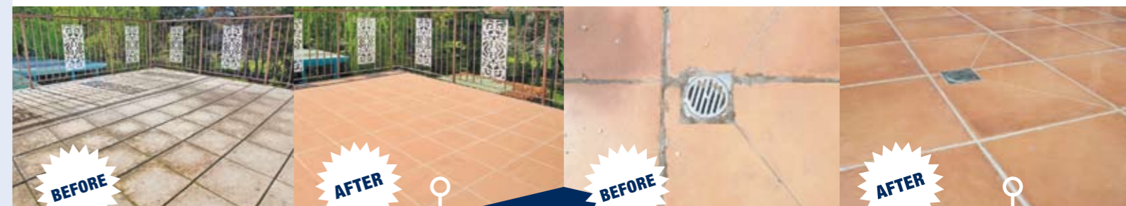
Tile over existing tiles
