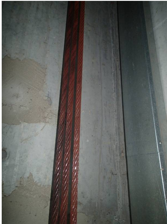
Rusty hoisting ropes must be replaced
