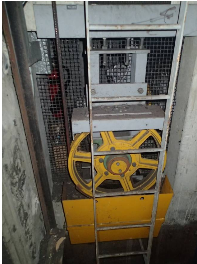
Hoisting machine oil leaks must be repaired and oily rags removed
