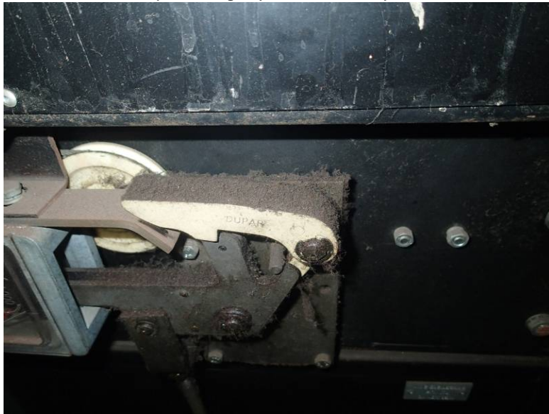
All lift shaft equipment must be cleaned
